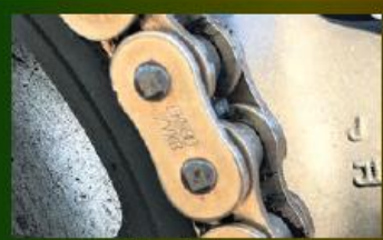
no rust, good condition
